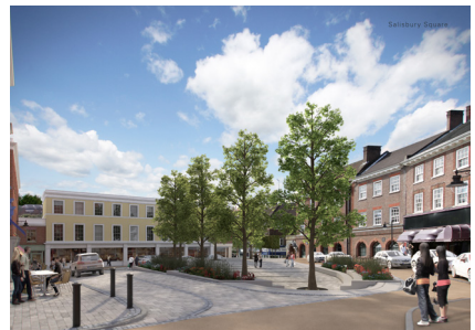
Above: The successful redevelopment of Hatfield Station.
